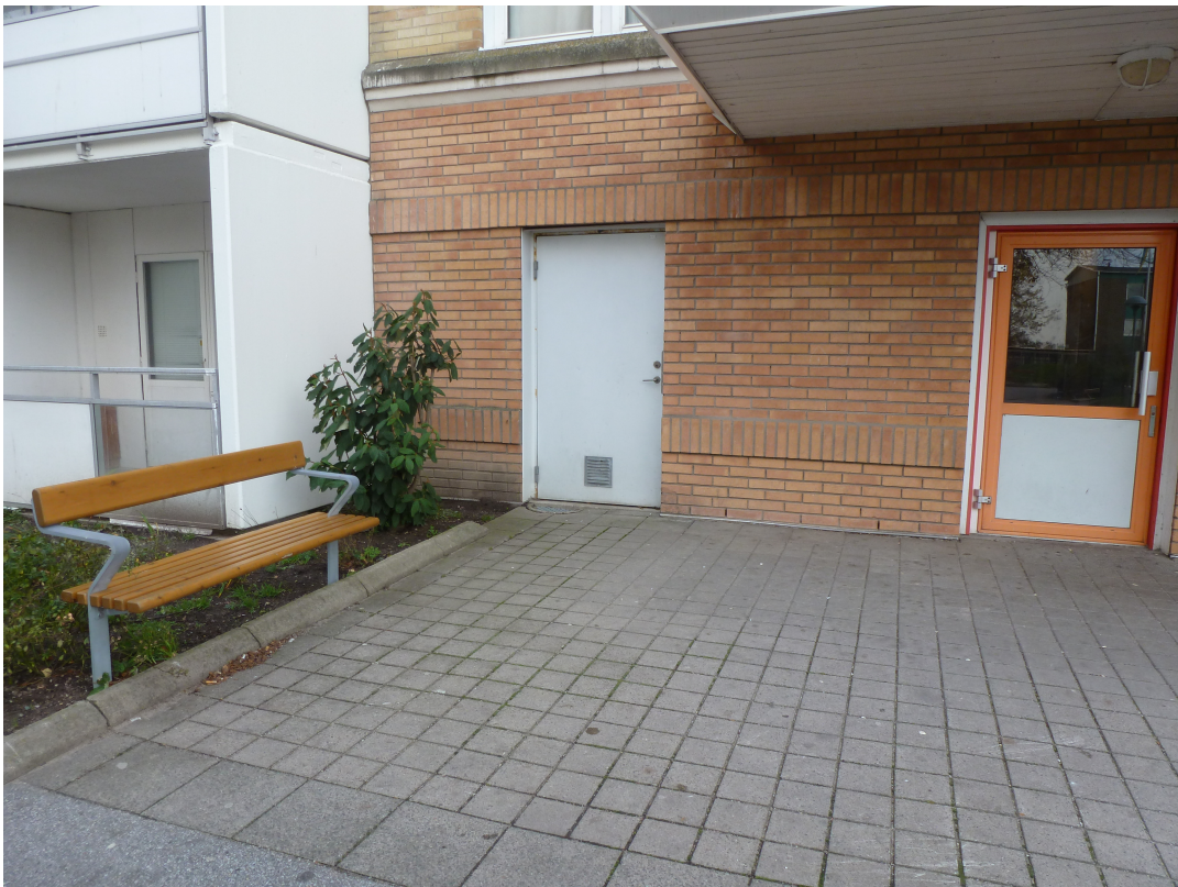
Figure 2: Park bench outside the front door of an apartment building without covering.
