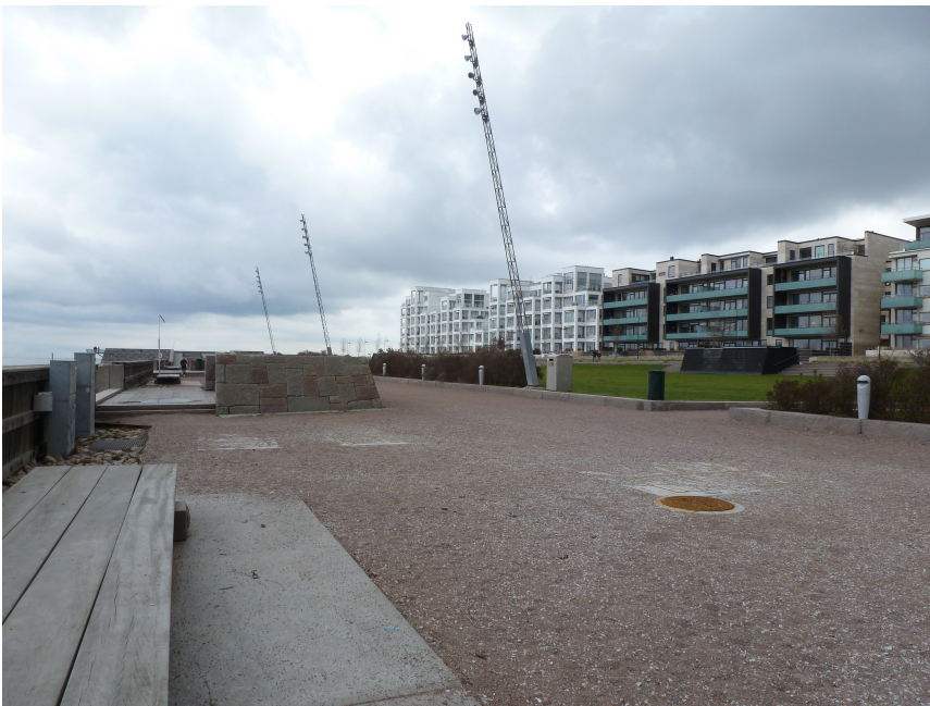
Figure 3: Wide view of main seating area in the Western Harbor.
